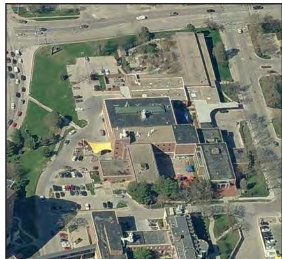
Figure 8-13 UNMC Provides Pervious Area around Buildings for Downspout Discharge
