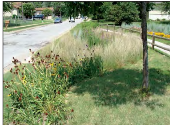
Figure 8-1 Structural BMP Application for Linear Roadway Project
