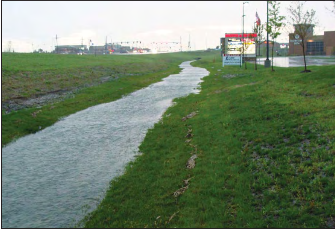
Figure 8-19 Bioswale
