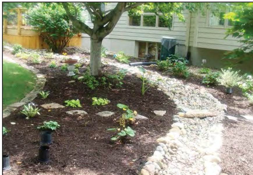
Figure 8-11 Example of a Downspout that is Disconnected from the Stormwater System
