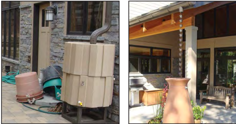
Figure 8-8 Examples of Residential Rain Barrels
