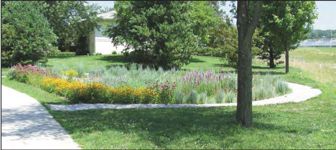
Figure 8-14 Orchard Park Bioretention System in Omaha, Nebraska
