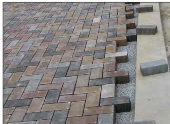
Figure 8-33 Example of a Permeable Paver Installation
