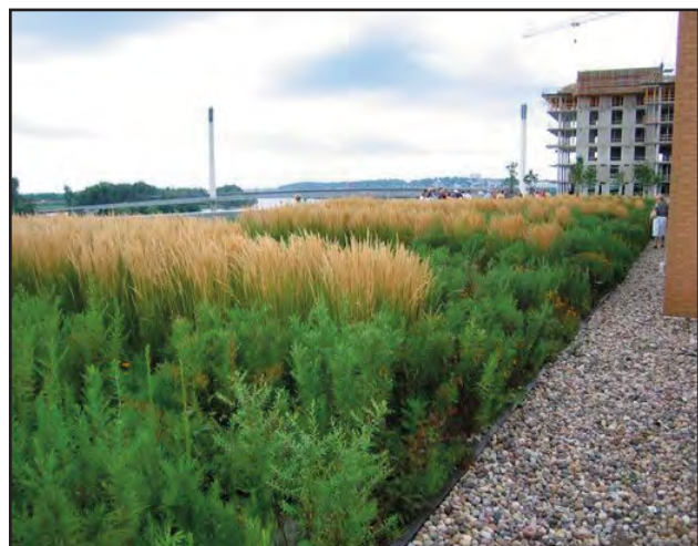
Figure 8-27 Gallup Campus Green Roof, Omaha, Nebraska ( www.omahaice.org )
