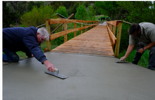
Roy Bailey and Dru DeLaet put the finishing touches on a new impact pad for the refurbished creek bridge. May 23, 2024. Photo by John P. DeLong.
