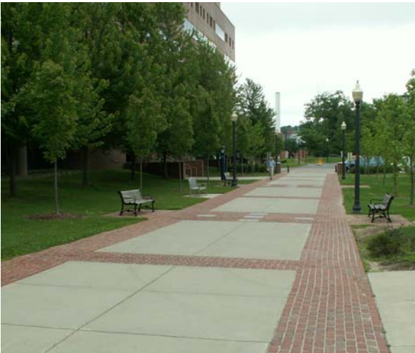
Scored concrete infill and brick edging (Penn State University)
