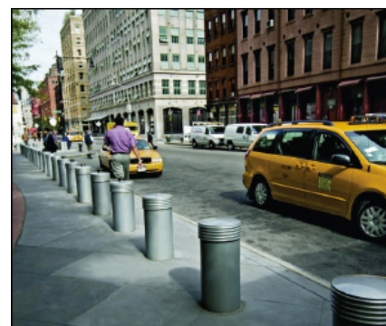
12" BOLLARDS — EMBED OR REMOVABLE. CAN HAVE LOW LEVEL LIGHT FOR REFLECTOR TYPE
