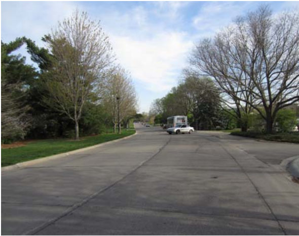
EXISTING: The Loop Road is curbed with standard catch basins
