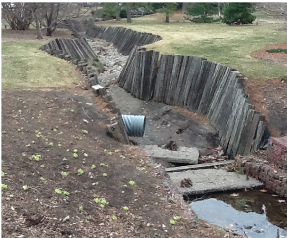
Drainage channel in Maxwell Arobertum
