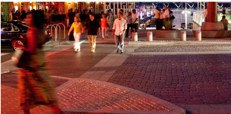
Stone pavements help to create a sense of place at a gateway (National Harbor, Maryland)
