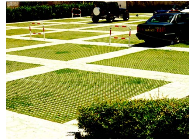
Porous paving installation
