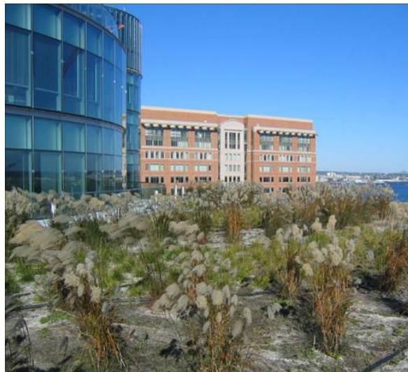
Green roof installation in Boston, Massachusetts
