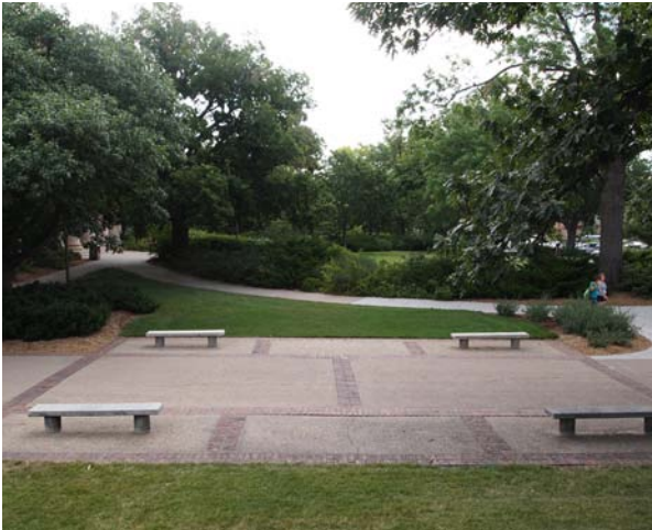
Exposed aggregate concrete and brick paving on 12th Street Mall
