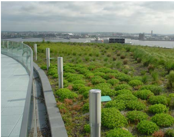
Green roof installation
