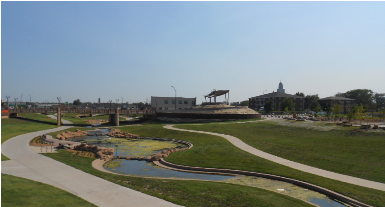
Recent improvements to Antelope Creek
