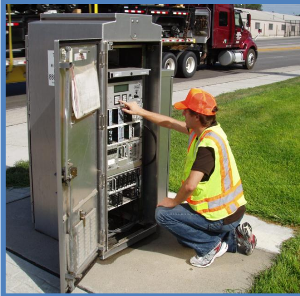
Fig. 2. Working on a traffic signal control box in Columbus, NE.
