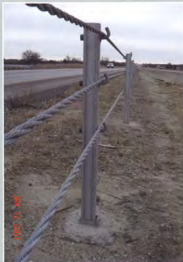
High-tension cable and guardrails.
