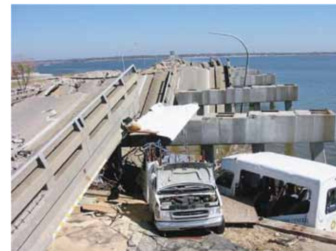
Bridge Hydraulics - US 90 - Biloxi (2005)
