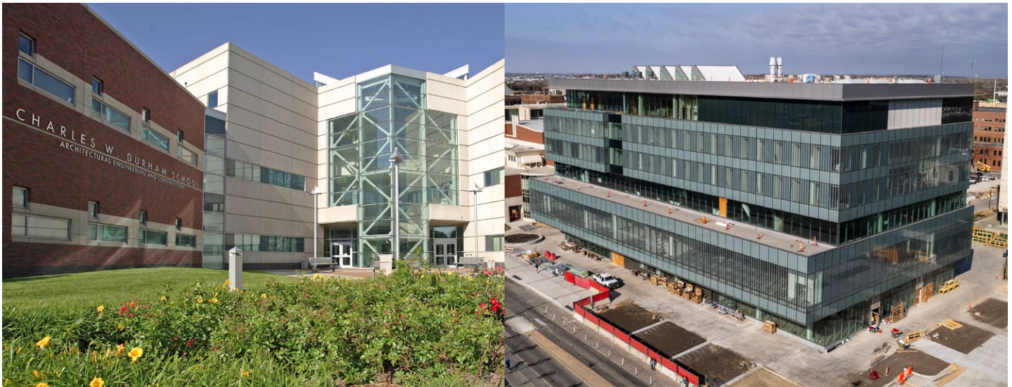
The Peter Kiewit Institute UNO Scott Campus Omaha, NE
