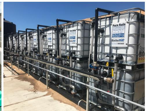
Stand alone filter system to filter metals from industrial sites. Photo by Ryan Holmann, Stormwater Biochar; filters by BioLogical Carbon
